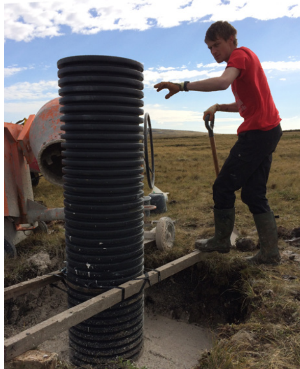
Figure 1 Installing a non-magnetic housing for the variometer at the Port Stanley test site.
