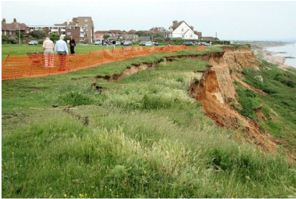
Figure 3 View of the new cliff-top landslide site at Barton on Sea, Hampshire, UK. This is an active landslide posing significant risks to the public and near-by infrastructure and buildings.
