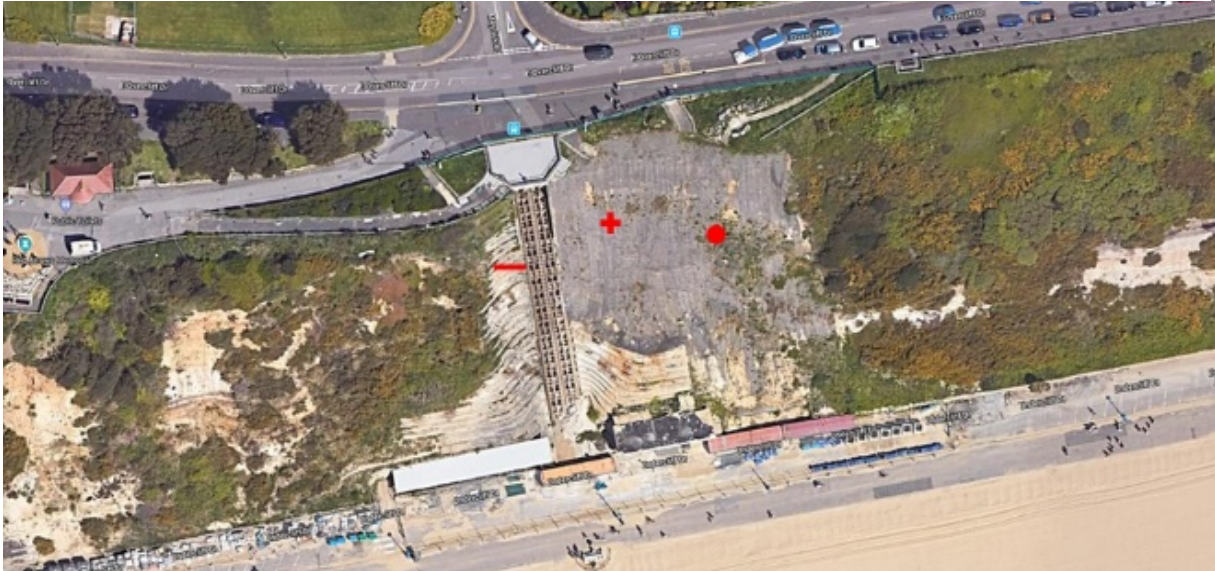
Figure 11 Aerial view of the landslide site East Cliff, Bournemouth, UK. Red symbols denote the deployment locations of the devices (symbols are also used to identify each device). One device (denoted by circle) is deployed on a mild slope; another one (denoted by cross) on a steeper slope; while the third one (denoted by dash) is deployed on the stone-paved support structure.
