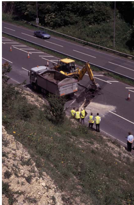
Figure 2. Excavation of fissure across north-bound carriageway of A 690, 20 June 2003.
