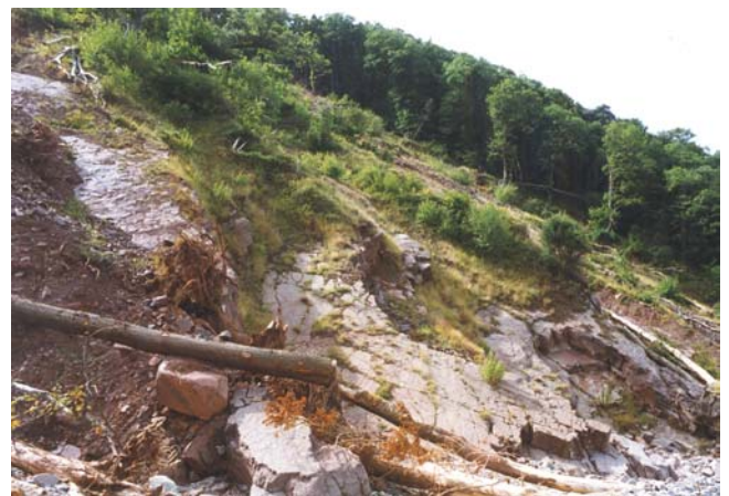
Figure 1 Well-jointed and bedded rock masses at Gore Point, near Porlock Weir lead to structurally controlled block slides where the dip of the discontinuities coincides with a slope.
