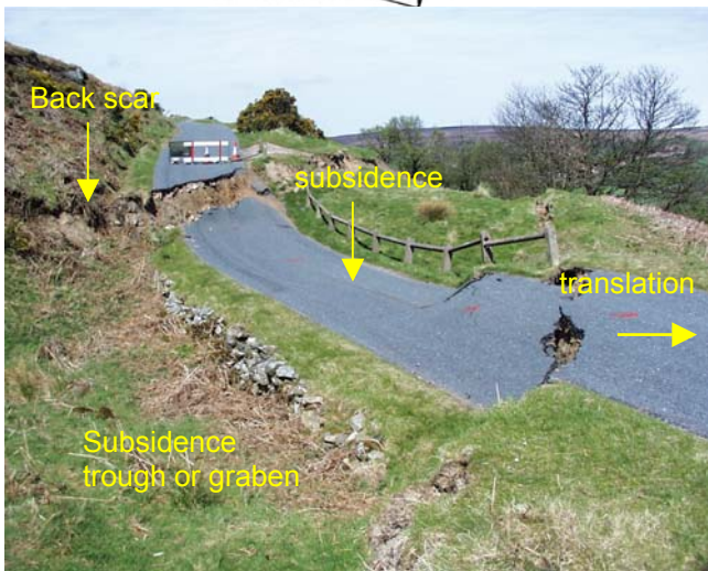
Figure 5 Where slides are non circular and have a translational element ground may subside into the void created between the backscar and the translated mass to create a subsidence trough or graben.
