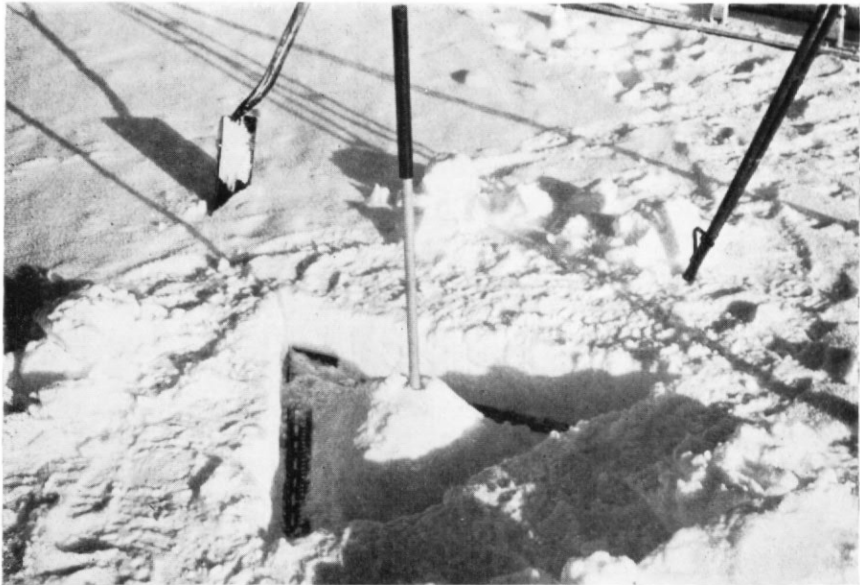
Fig. 3. The emplacement of the portable Dexion frame which was used as a base for the theodolite tripod.
