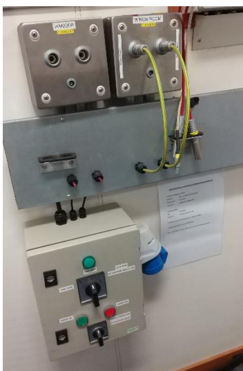
Changeover switch with 230V supply and earth for cable discharge.
