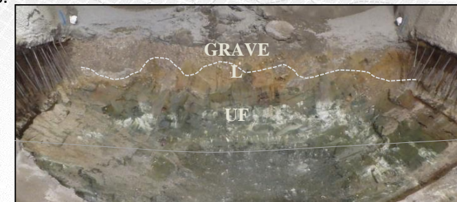
CH1 Pilot Tunnel
