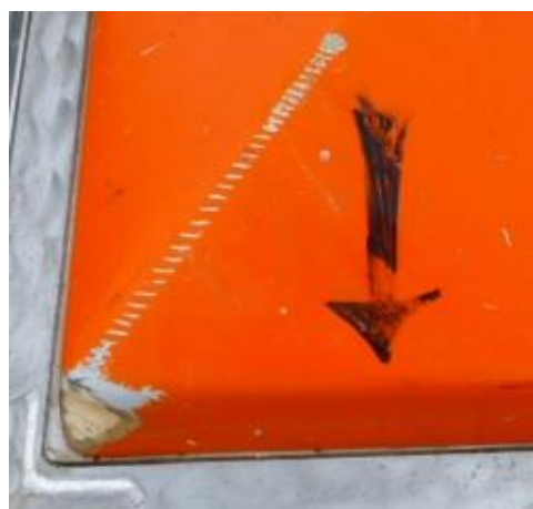
Figure 25: Trawl wire damage to frame
