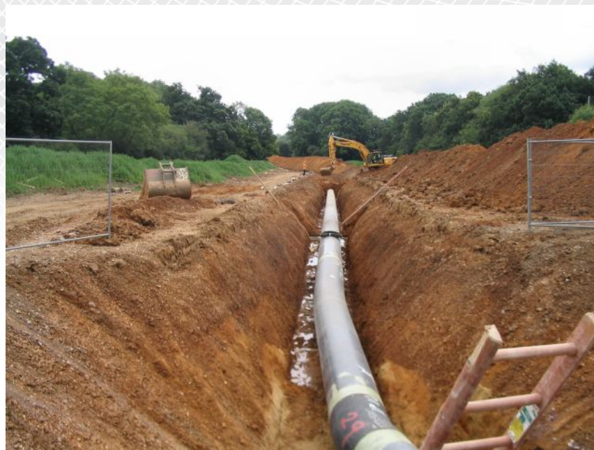
Rosemary Oakeshott - Gas pipeline internment CC BY-SA 2.0
