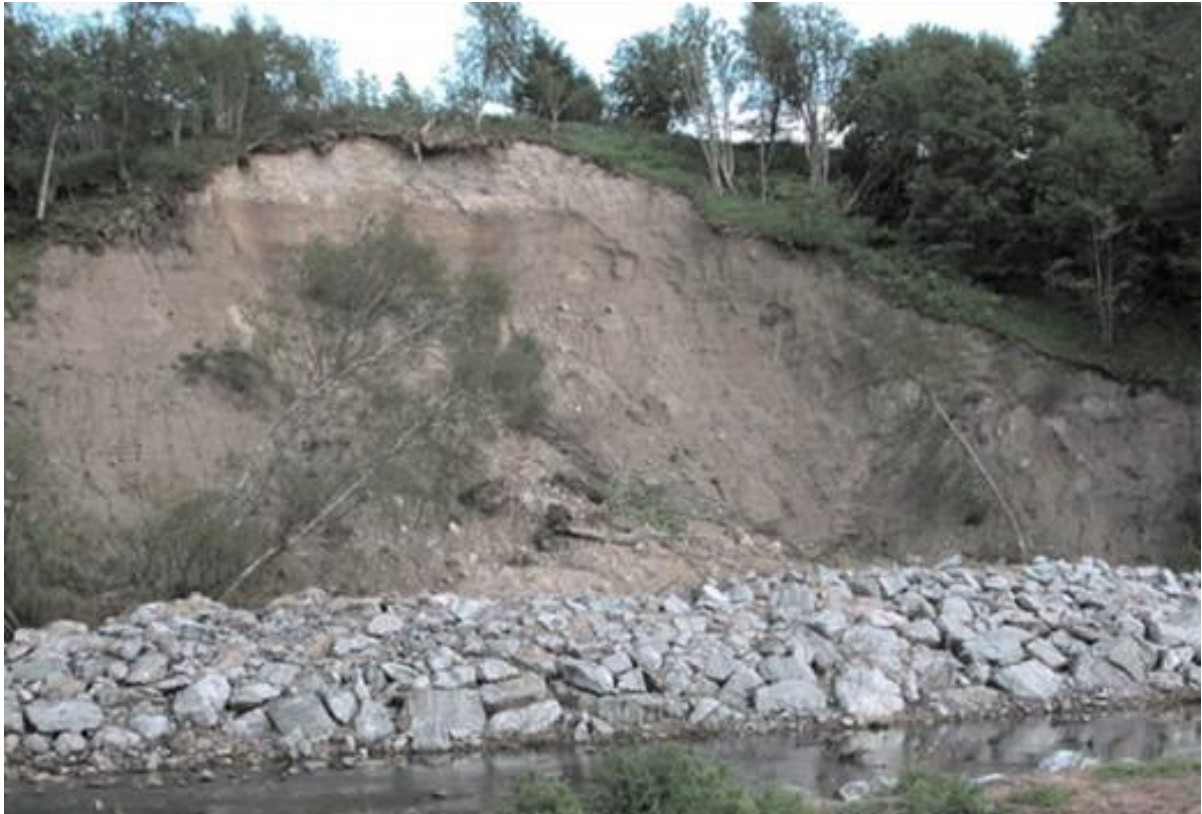
Figure 129. The Dulnain Bridge landslip section in June 2003, looking south.
