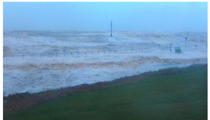
Figure 2. The Crosby sea wall frontage, 5 December 2013. Photo provided by the Sefton Council.
