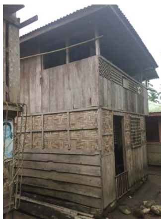
Figure 5. Example house from Plaridel showing timber façade, hipped roof, and concrete slab base.
