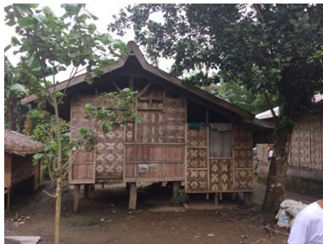
Figure 4. Example house from Calabnian showing woven palm façade, roof level ventilation, raised ground floor, and sunken post foundations.
