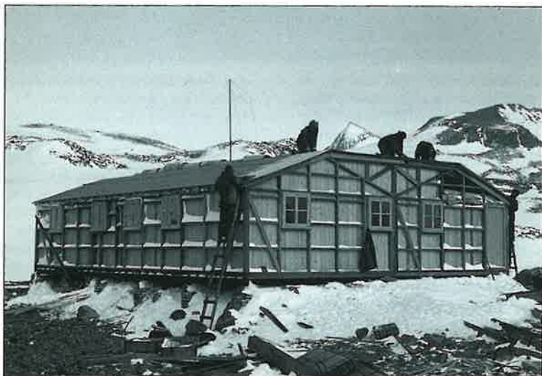
Constructing Hope Bay hut, 1945.
