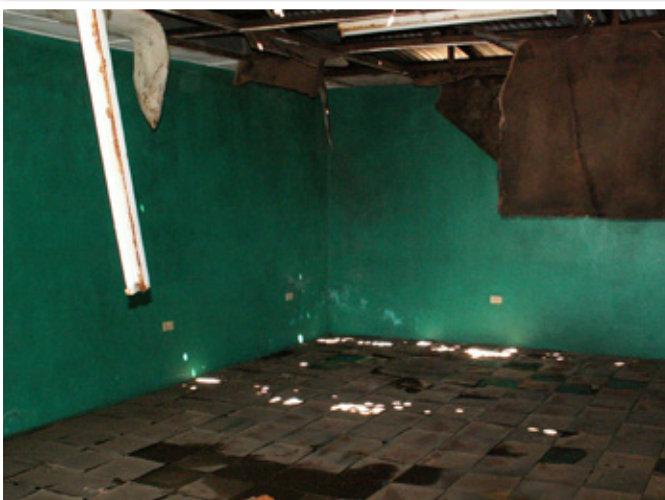
LGS office (December 2013).
