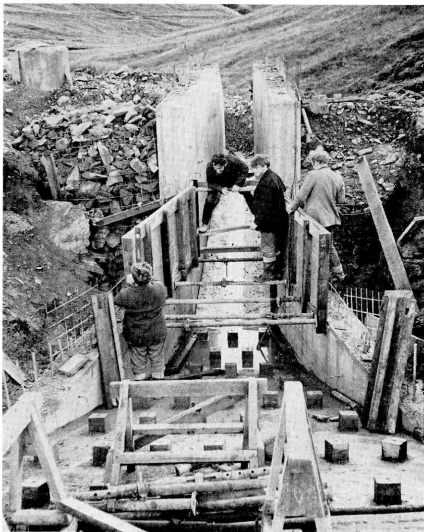
Figure 1 Steep stream gauging structure under construction at Plynlimon
