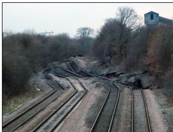
Figure 1: Network Rail tracks affected by Hatfield Colliery landslide. Photograph taken 23 rd February 2013. T. Dijkstra ©NERC
