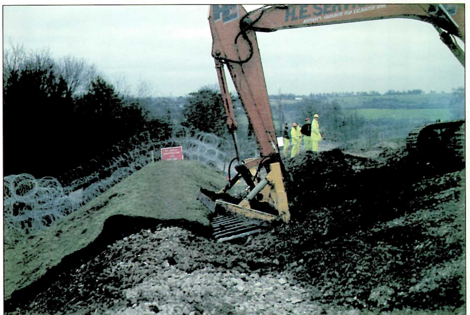
Plate 18. Macro-turfing machinery in action
