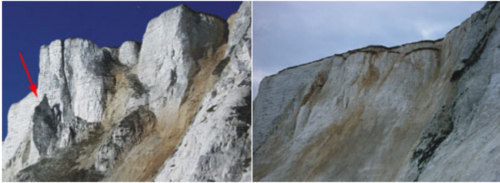
Devil's Chimney before (left) and after (right) the landslide.
