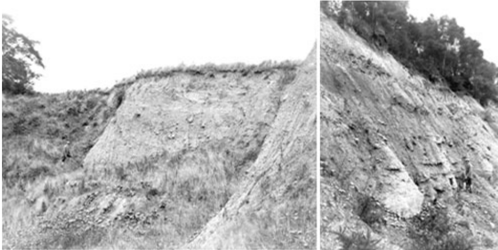
Figure 6 The backscarp of Lloyd's Coppice landslide from 1924
