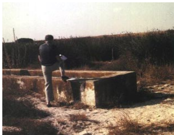
Old cattle watering trough in the Doñana national park, southern Spain, previously fed by a flowing well but now abandoned due to piezometric level drawdown after intensive development in nearby areas. Water discharged was fresh palaeowater.
