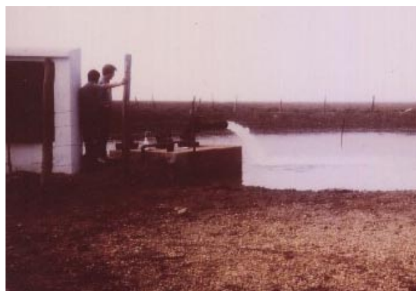
A pumped well discharging palaeowater to sustain the impoundment of a lagoon used by waterfowl in the dry season. Doñana national park, southern Spain.
