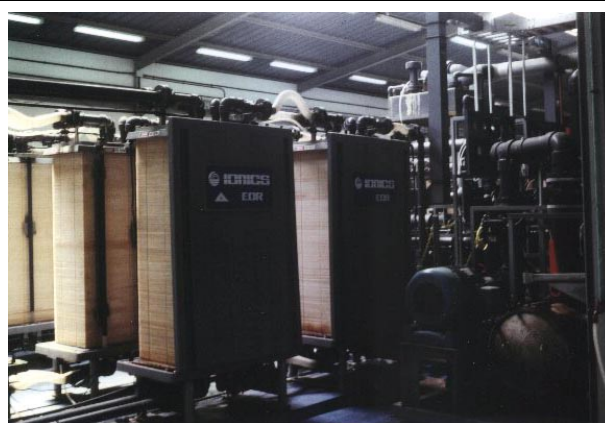
Electrodiagnosis plant in Playa del Ingles, Gran Canaria, to desalinate brackish palaeowater
