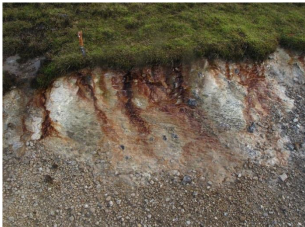
downslope edge of limestone spoil heap
