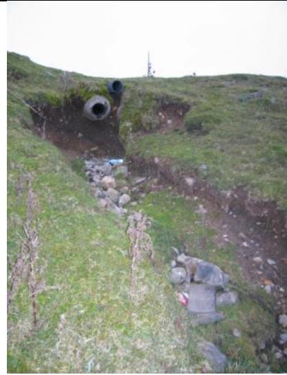
Road drain that likely contributes to spring flows during periods of high rainfall (upper part of site)
