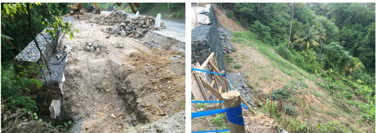
Figure 16 Landslide stabilisation works along the Vieux Fort-Castries road at Thomazo.
