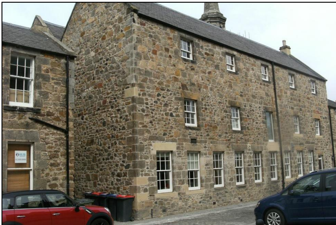
Photo ELC_12 P1: The building which houses the John Gray Centre in the middle of Haddington contains blocks of porphyritic trachyte, probably from Peppercraig Quarry. © BGS, NERC.
