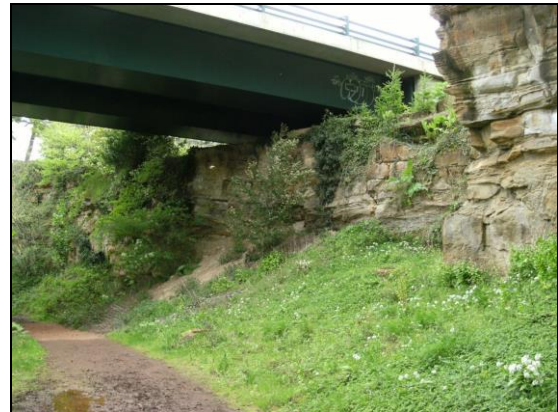
Photo ELC_17 P7: Cliff section continues along the east bank of the River Esk and has been used as a foundation for the A68 which crosses the river at this point. © BGS, NERC.
