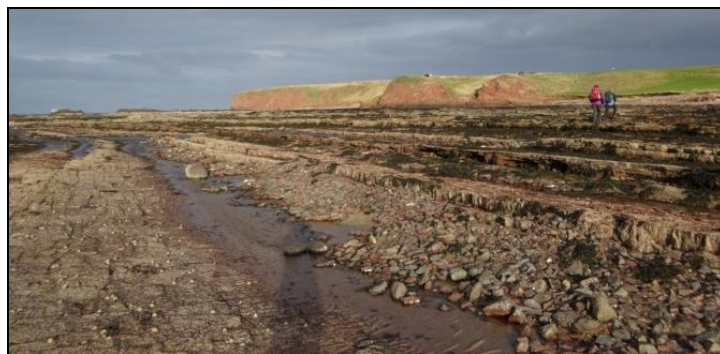
Photo ELC_4 P3: View looking east across the bay north of Winterfield Golf Course, displaying gently dipping strata belonging to the Ballagan Formation of early Carboniferous age. The sequence is made up of interbedded mudstones and cementstones, dissected by numerous faults and igneous intrusions (vents and dykes). © BGS, NERC.
