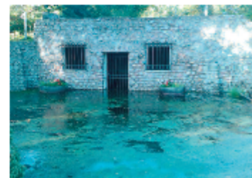
Taffs Well in 2010. The well building was flooded, access was unsafe and the doors had been shut for most of the previous 50 years.
