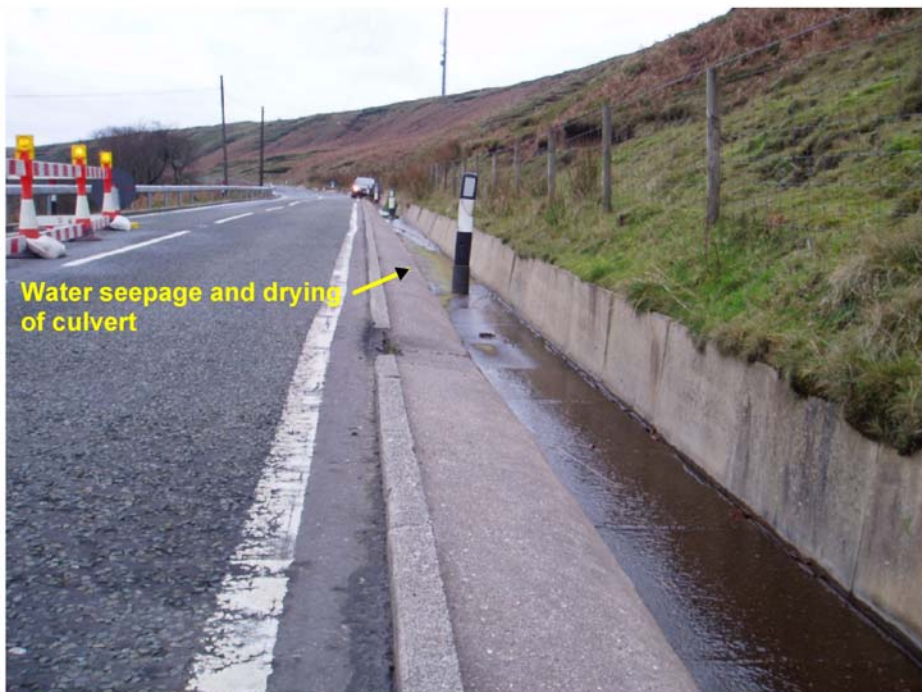
Figure 3-5. View of the drainage culvert immediately behind the Little Hey landslide. Photograph taken from [BNG 409865 404414], facing 240° (SW) (H.J. Reeves, BGS © NERC 2004).
