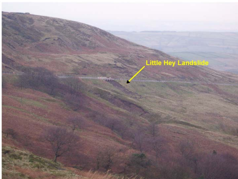
Figure 3-1. View close-up of Little Hey landslide taken from [BNG 409821 403950], facing 002° (N) (H.J. Reeves, BGS © NERC 2004)
