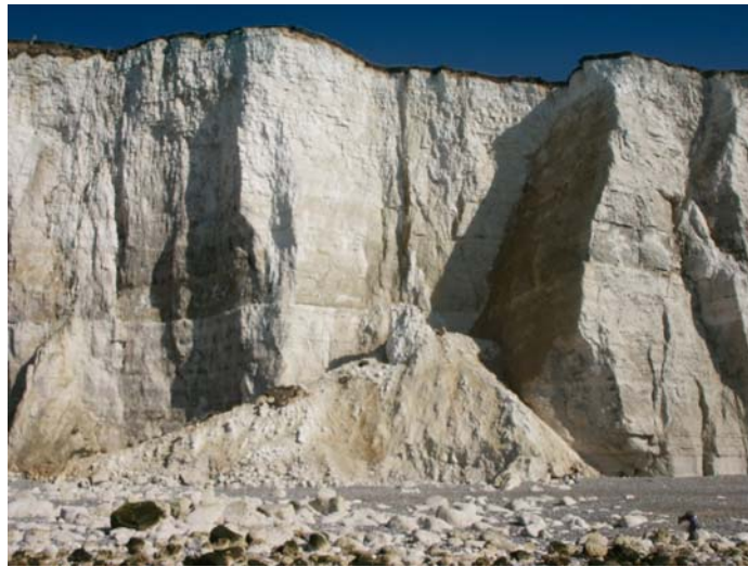
Figure 6.19. Collapse naturally controlled by West dipping master joints, Puys, France.
