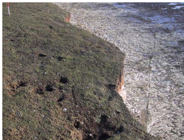
Figure 6.2. Large fracture developing in the cliff top at the Birling Gap research site. Also note the fault running along the wave cut platform that intersects the research site.
