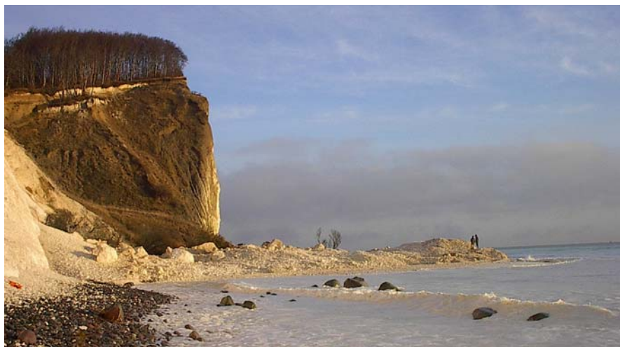
Figure 6.6. Cliff collapse at Jättebrinken in January 2004.
