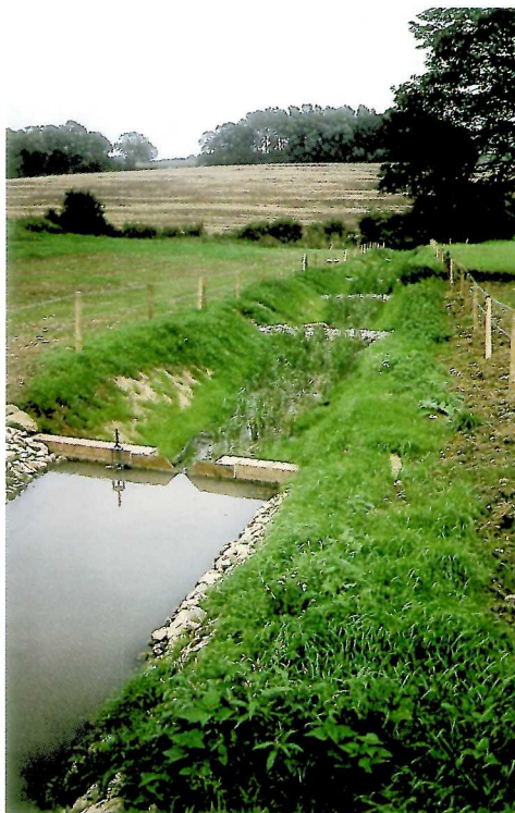
Plate 18. A farm sewer dyke used to clean wastewater before it is discharged into a local stream. The dyke is shown eight weeks after planting with reed seedlings (Severn Trent Water Authority)
