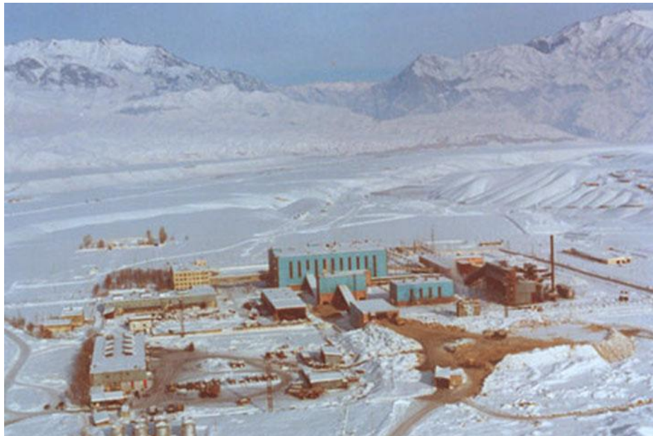
Figure 8 Different views of the processing plant
