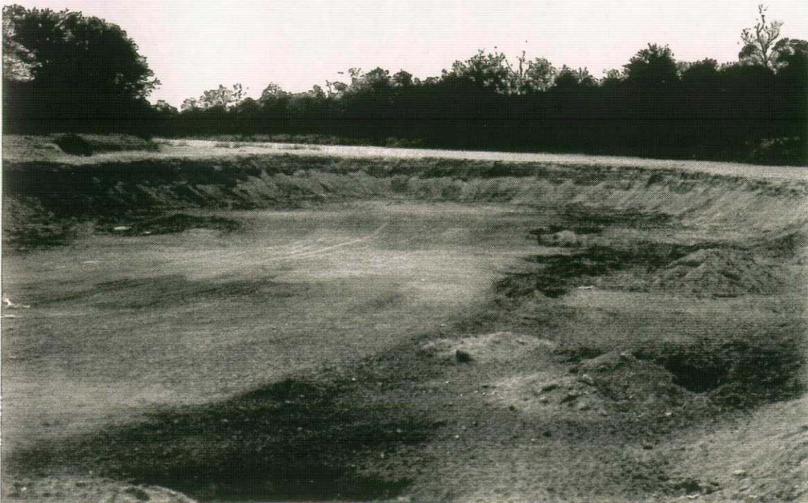
Figure 7 Masunga sand pit excavated into the bed of the Tati sand river to the top of the basal saturated zone.
