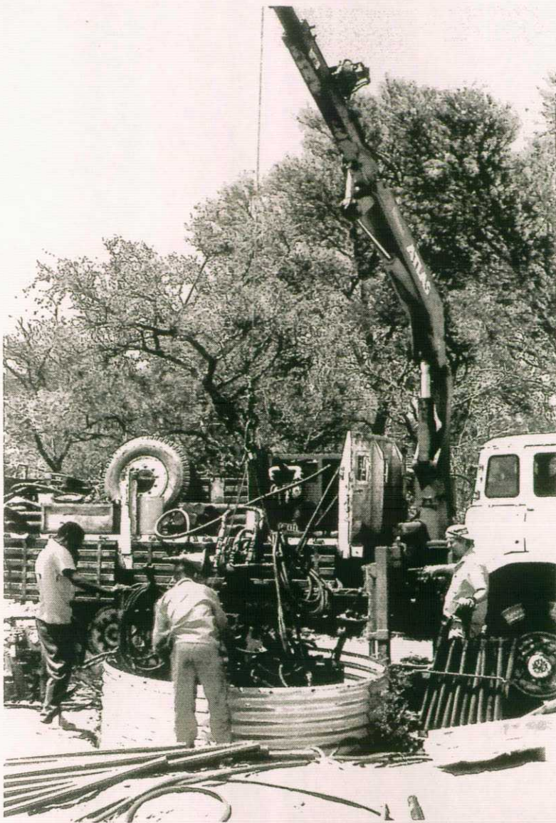
Figure 11 Emplacement of lateral drilling equipment at Masunga site A
