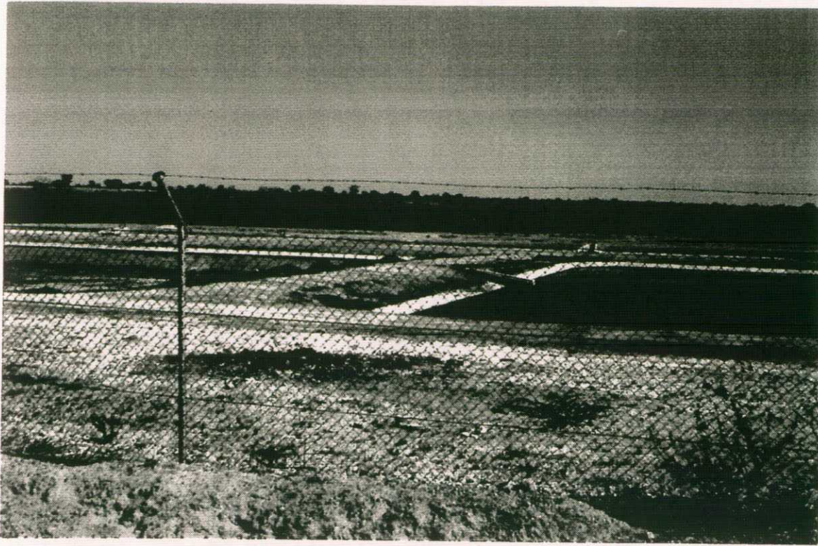
Figure 16 Sewage water treatment plant located adjacent to the Tati River upstream of Masunga site B.
