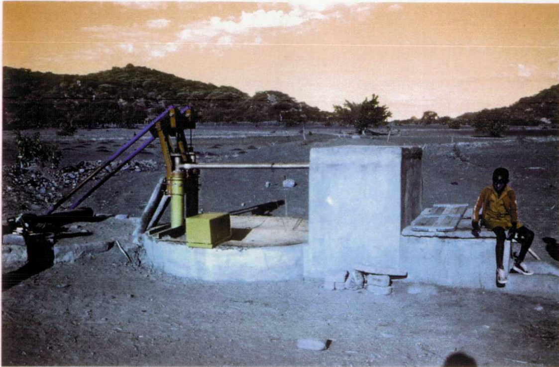
Figure 10. View of well completion showing two Bush pumps, well cover, water level recorder, header tank and meter box.
