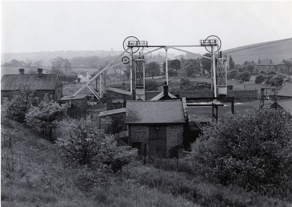
Brinsley Colliery looking south. This picture, by an unknown photographer, was probably taken shortly before the headstocks were dismantled in the first week of June 1970. The building on the far left contained the winding engine. During the making of the film Sons and Lovers (1959–60) the headstocks were painted a light blue colour to make them stand out. Eastwood church is just visible on the skyline. (Photo: British Geological Survey archives, P711164)
