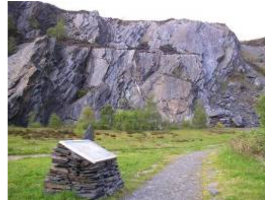
FIG. 2. Ballachulish Slate Quarries opened in the late-17th century and continued to operate until 1955. Today the area is enjoyed by the local community and visitors, with a prepared path and information boards interpreting the geology and industrial heritage. (Photo: John Gordon).
