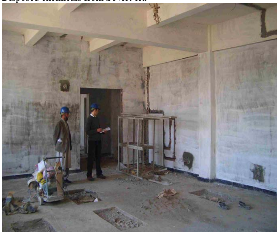
Sample Preparation laboratory under refurbishment
