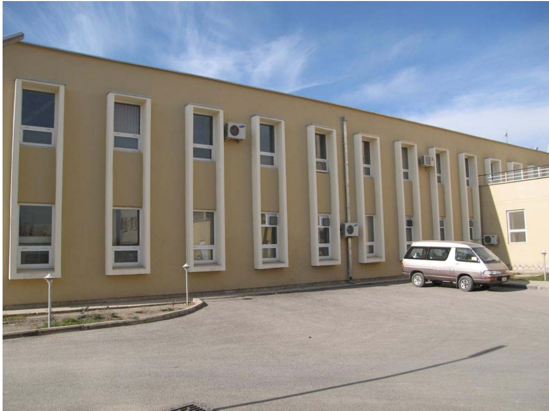
Refurbished Annex building (June 2006)
