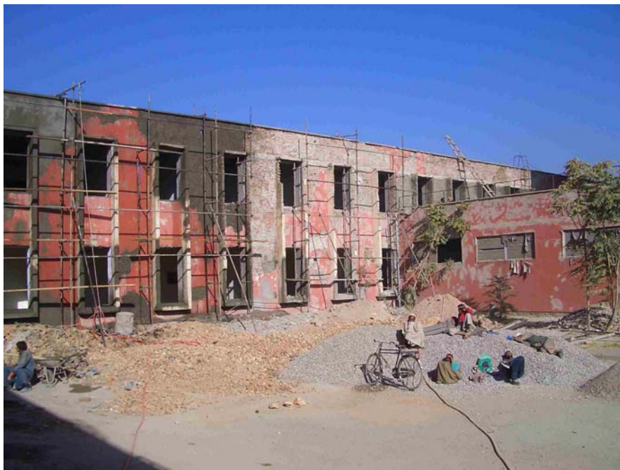
AGS Annex building – laboratories (under refurbishment Feb 2006)
