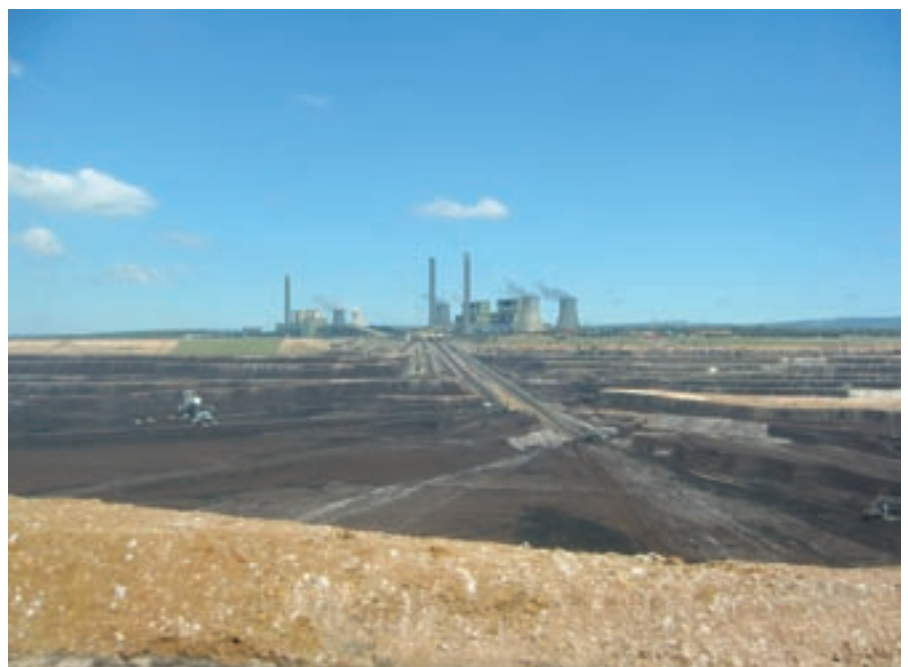
CO 2 capture and storage (CCS) is the only the way to achieve near zero emissions from coal-burning power plants, such as these in the Latrobe Valley, Australia.
