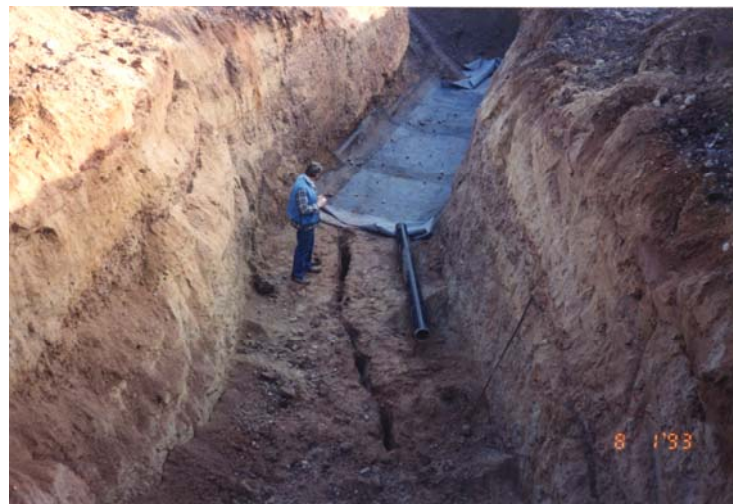
Figure 7. Faults that have reactivated contemporaneous with mining, seen exposed in an inspection trench. (A) The fault plane is clearly visible having displaced the superficial deposits and dilated the plane to produce a fissure, up to 1 m wide and several hundreds of metres long. The back wall of the exploratory trench shows the horizontal displacement of the fault plane, which was subsequently infilled with red-brown granular soil and vertical displacement of a pebble bed horizon in the Sherwood Sandstone Formation. (B) Geotextile grids were deployed to mitigate against further movements along the fault, Downes Bank, Oulton, Staffordshire (after Donnelly 1994).
