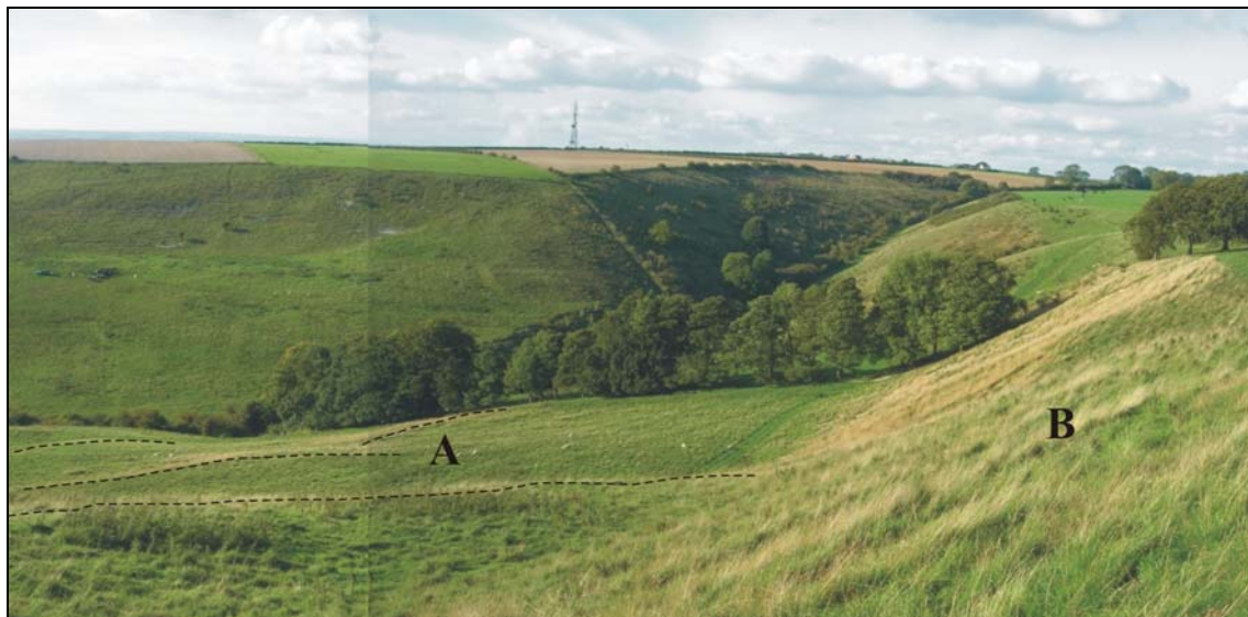
Figure 24. A view of the Back Warren Plantation landslide taken from NGR 480024 461270, orientation 335° (NW). A: Rotated blocks, B: Back scar.
