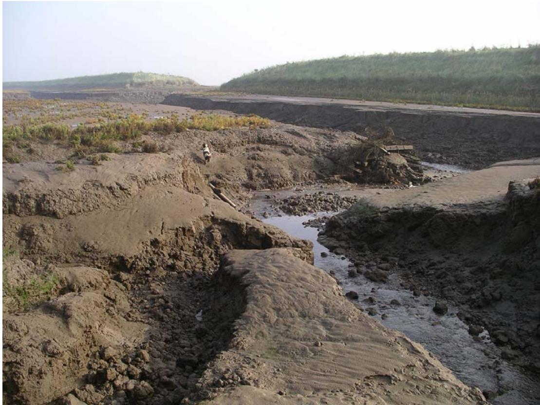
Photo 9. 6. New creek running into soke dyke behind the old embankment, looking towards central breach. Photo: Sue Brown, October 2005
