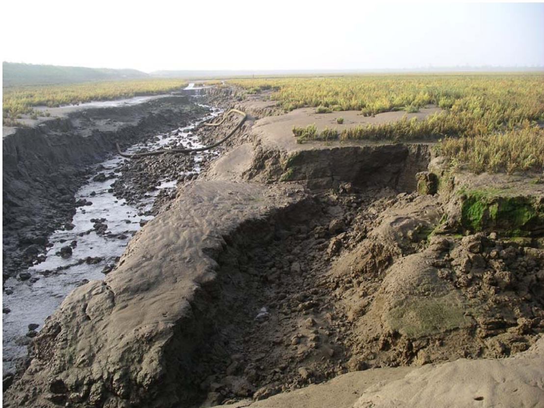
Photo 9.9. New creek (shown in 9.6) cutting back towards TDS6, looking away from central breach. Photo: Sue Brown, October 2005
