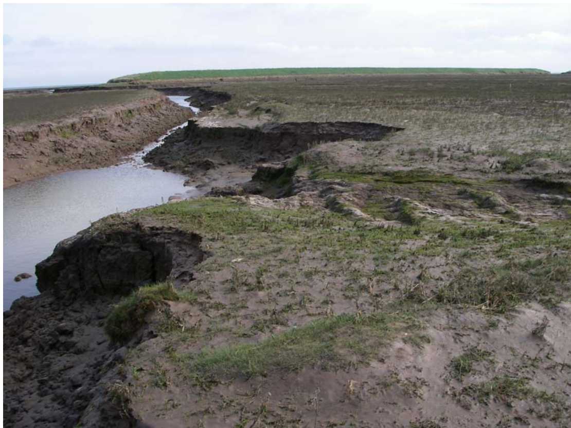
Photo 9.5 Creek side erosion of excavated creek inside MR, looking towards central breach. Photo: Sue Brown, April 2007
