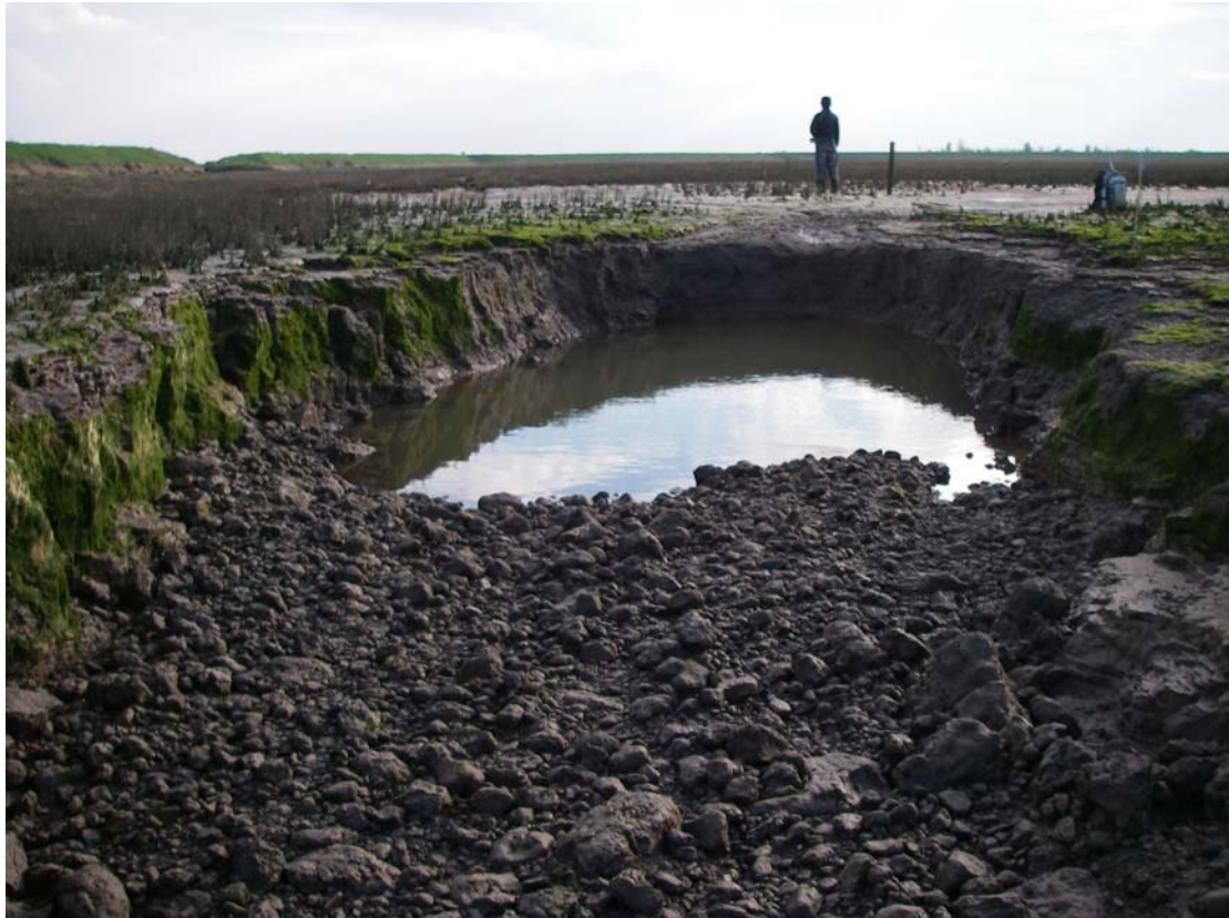
Photo 9.12. Headward extension of new creek (shown in Photos 9.9-9.11) now close to TDS6 (figure standing at TDS6). Photo: Sue Brown, April 2007
