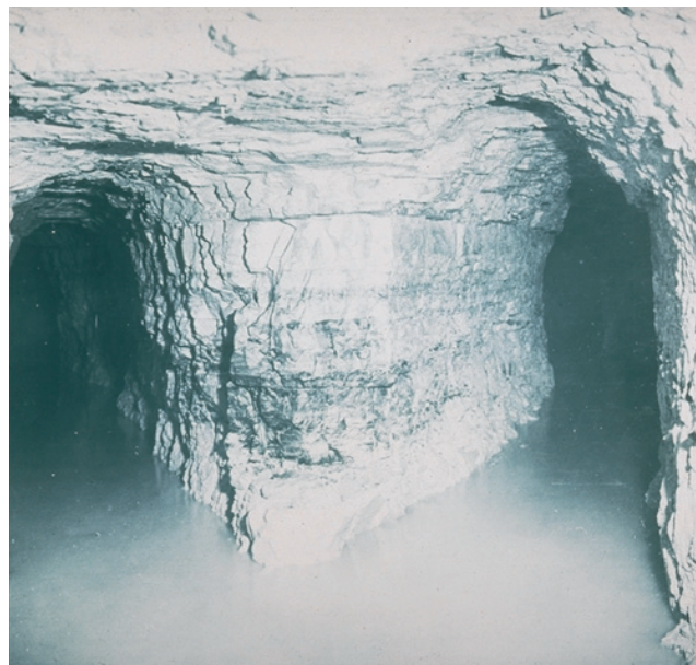
Plate 3 Converging adits in the Cottingham shaft and adit source (Courtesy of Yorkshire Water Services plc).
