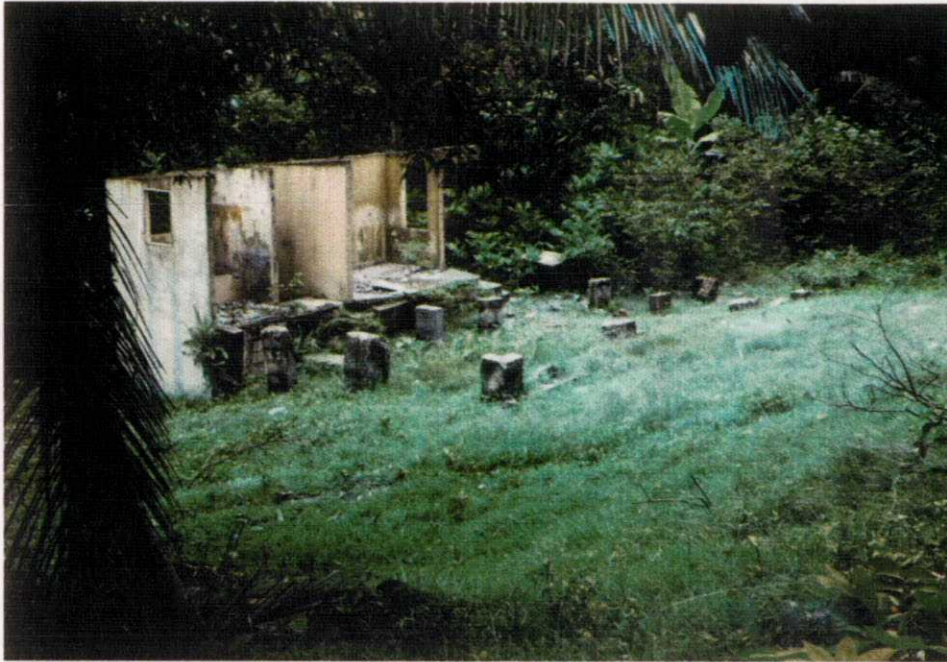
Figure 3.10 Toe zone of a medium-sized rotational landslide that caused destruction and abandonment of a house in 1986 at Ivy Store, near Cross Roads, 1km south of Chapelton.. The slide has occurred downslope of the main road in a clay regolith (Nonsuch Clay) overlying weathered strata of the Yellow Limestone Group (probably red clay and fine grained clastic sediments).
