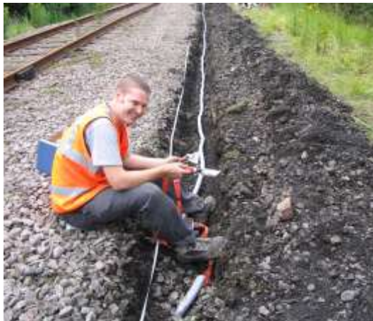
a. Retro-fitting electrode arrays for electrical resistivity imaging.
