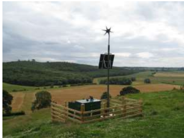
b. Field instrumentation cabin powered by renewable energy.
