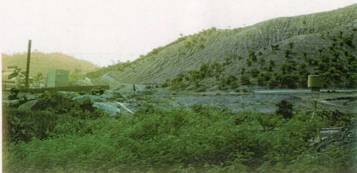
Plate 2.1. Obuasi mine complex and the ore-roasting chimney. Hill slopes to the north of the chimney (prevailing wind direction) have been stripped bare of vegetation by historic atmospheric emissions of arsenic trioxide (and sulphur dioxide) from the plant.
