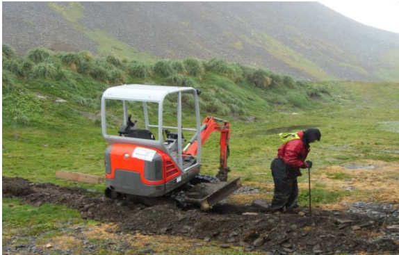
Cable trench digging at King Edward Point, South Georgia
