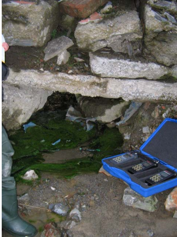
Figure 3.6 The culvert [SN 723 741]
