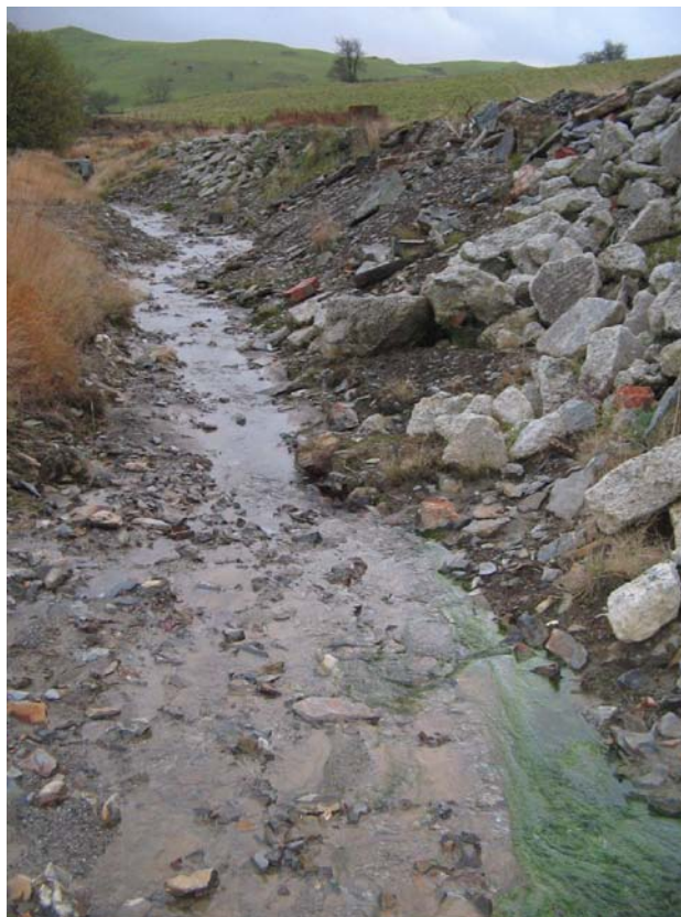
Figure 3.7 Frongoch stream immediately downstream the culvert
