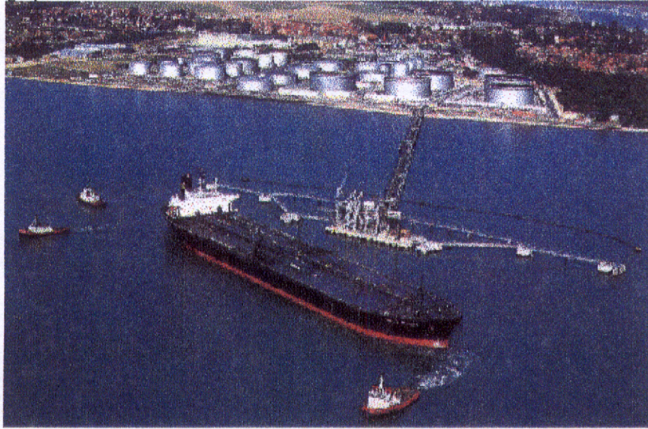
Figure 4.2 Aerial photograph of the BP Oil Terminal at Hamble on Southampton Water.
