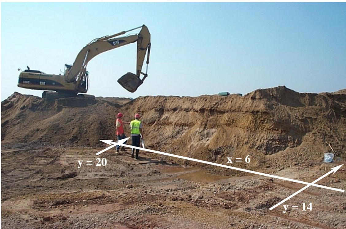
Figure 12. Excavation of the ‘5 m bench’, approximately along the line  $x = 6$ , between  $y = 14$  and  $20$ . The hummocky surface of the Mercia Mudstone shallows towards the bottom of the grid, as seen in the GPR 100 MHz data.
