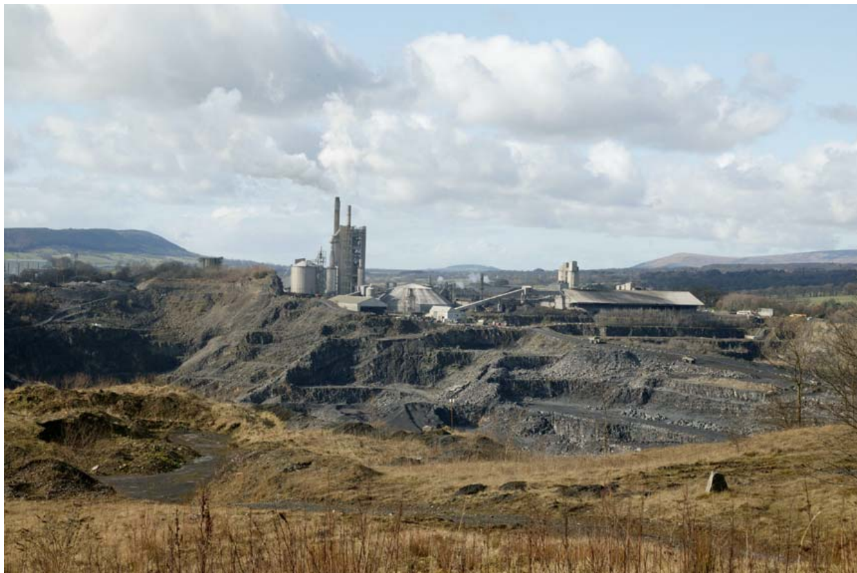
Figure 4. A view of Lanehead Quarry and the Ribblesdale Cement Works, from the nearby village of Chatburn. Quarry is working the Carboniferous Chatburn Limestone. Photo Courtesy of Castle Cement Ltd
