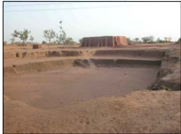
Topsoil from agricultural lands is removed for brick making
