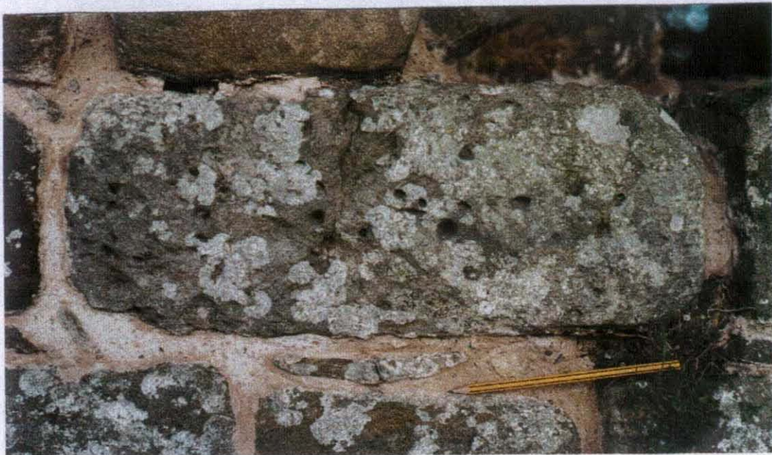
Figure 12. Outer face of south wall. Conspicuous hollows in Type 'B' stone, marking traces of fossil rootlets.
