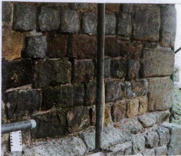
Figure 13. Outer face of north wall. Pale grey Type 'B' stone contrasts conspicuously with dull brown Type 'A' stone.
