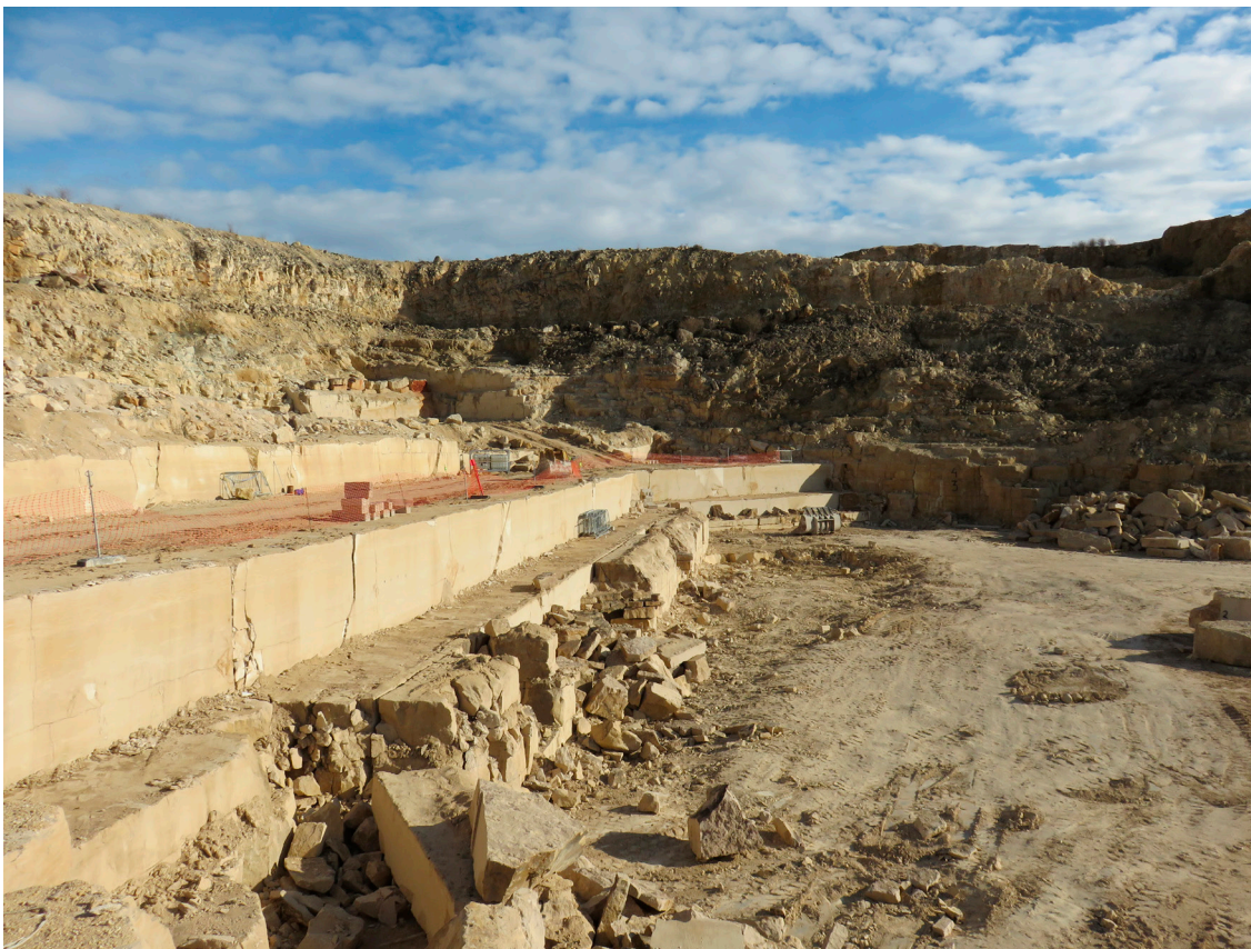
Cadeby Quarry, Doncaster, South Yorkshire, where beds of Permian dolomitic limestone are worked for building stone.
