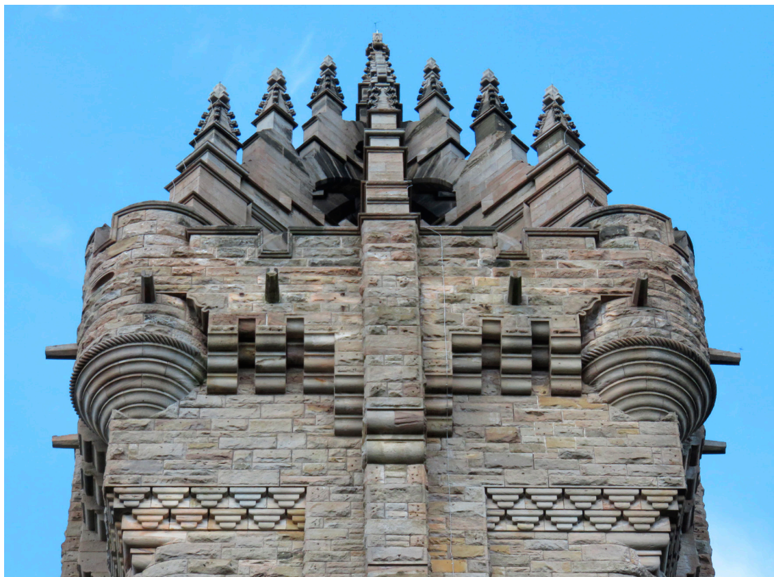
The National Wallace Monument, near Stirling, Central Scotland, constructed of Carboniferous sandstone quarried from the Abbey Craig on which the tower stands.
