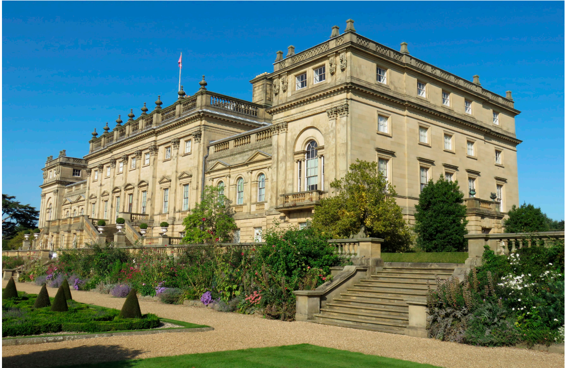
Harewood House, near Leeds, West Yorkshire, constructed of Carboniferous Millstone Grit sandstone.
