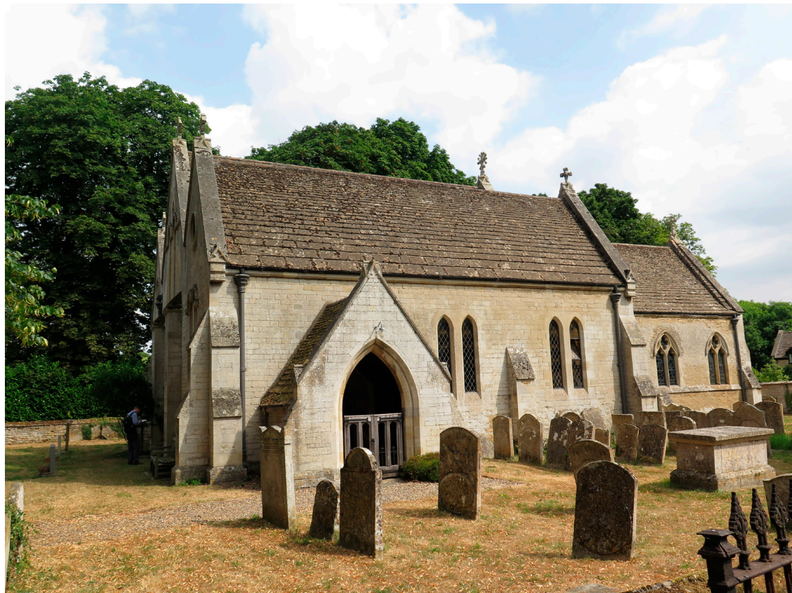
Church of St John the Baptist, Stibbington, Cambridgeshire, constructed of Middle Jurassic Lincolnshire Limestone.
