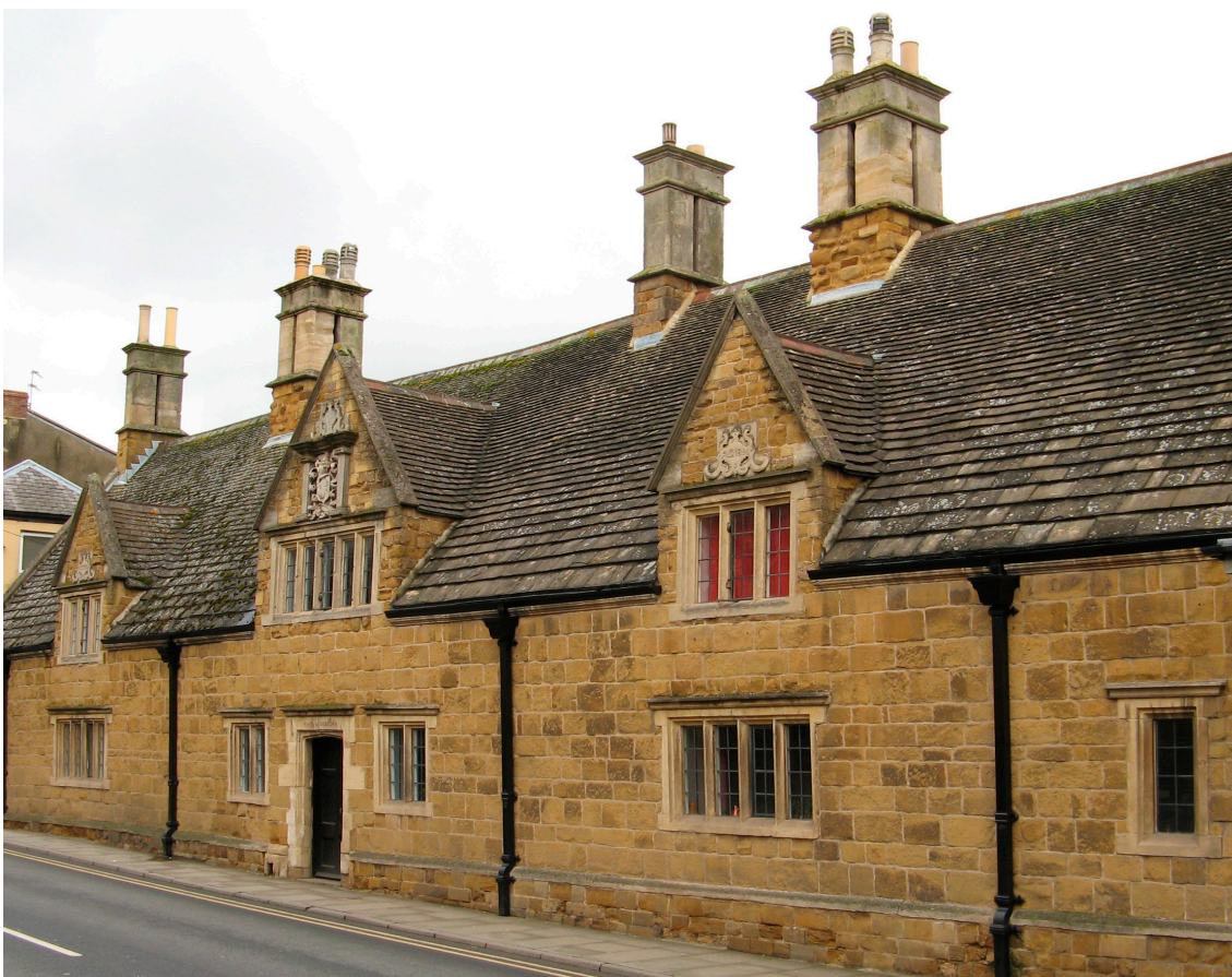
Maison Dieu Bedehouses, Melton Mowbray, Leicestershire, built of ferruginous limestone ('ironstone') and roofed with Collyweston Stone-slate (all of Jurassic age).
