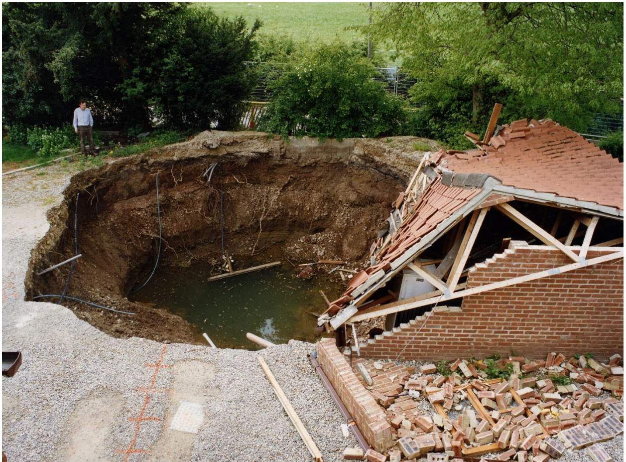
Figure 55. Sinkhole that formed in 1997 on Ure Bank, Ripon, destroying four garages and damaging the adjacent house. (Photo P. Tod © UKRI/BGS).
