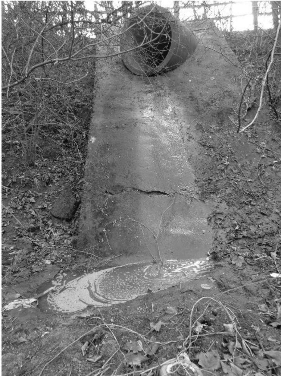
Figure 40. Motorway drainage pipe feeding Wadworth Wood Sink 5 (from Higgins, 2018). Photo courtesy of Mike Higgins.
